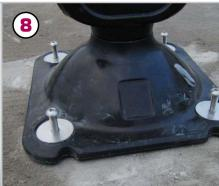
Position product centering the four holes. Remember to make sure the front of the bollard reach the threaded part of the Anchor. Make faces oncoming traffic. Place the large washers over the button head screws and place through the nylon inserts and into the Anchor.
