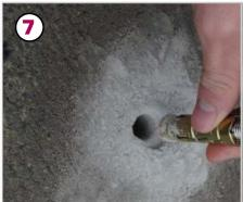
Screw the 100mm button head screws into the Position product centering the four holes. anchor shields so the thread end is just past the Remember to make sure the front of the bollard base of the anchor. Ease into the holes until the faces oncoming traffic. Place the large washers top of the anchor is flush with ground level. Tap lightly with a hammer if necessary.
