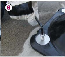
The fixing screws should drop down until they sure all four bolts are engaged in the shield thread by 2 or three turns then proceed to tighten all four bolts to torque setting 27.
