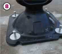
over the button head screws and place through the nylon inserts and into the Anchor.
