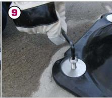
The fixing screws should drop down until they reach the threaded part of the shield. Make sure all four bolts are engaged in the shield thread by 2 or three turns then proceed to tighten all four bolts to torque setting 27.
